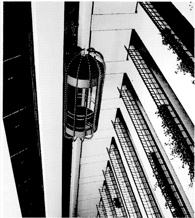
A modern elevator.
