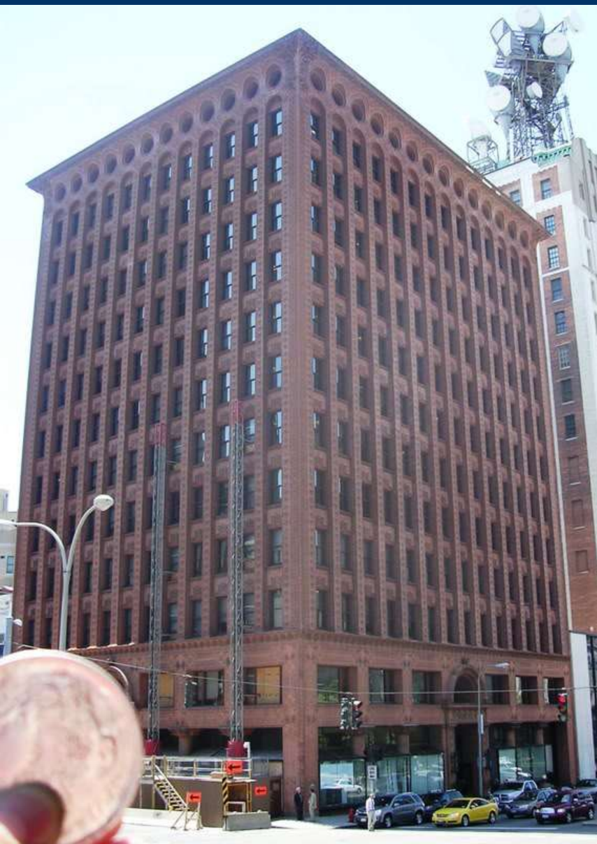
The division of the façade; base, piers, and attic is similar to classical columns.
