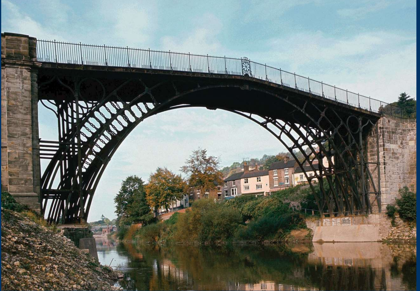
Abraham Darby III and Thomas F. Pritchard, Cast Iron Bridge at Coalbrookdale , England (first use of iron in bridge design. Strong and light material), 1776-79. 100' span.
