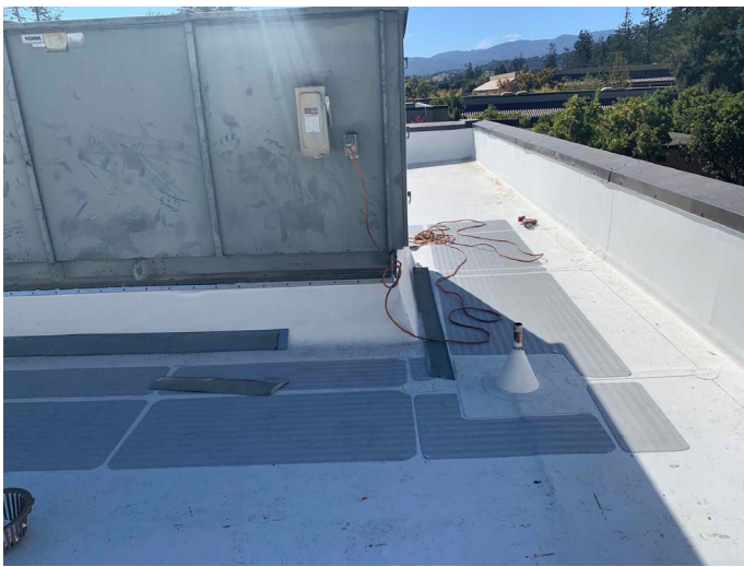
Example Photos of Singly Ply Upgrade
